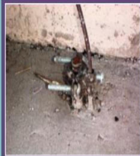
Improper Grounding
